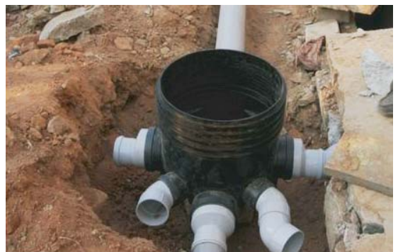
Simplified Sewer System - Individual house connections
