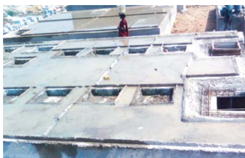
DEWATS during construction completion stage
