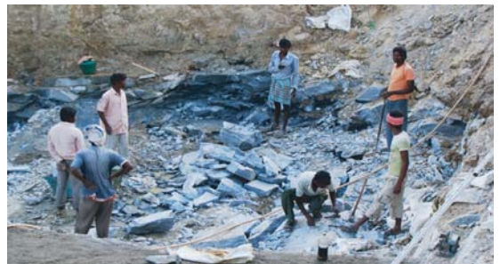
Rocky layer removed after blasting - Excavation stage
