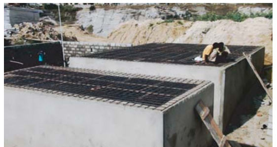
Construction stage - Top slab steel reinforcement
