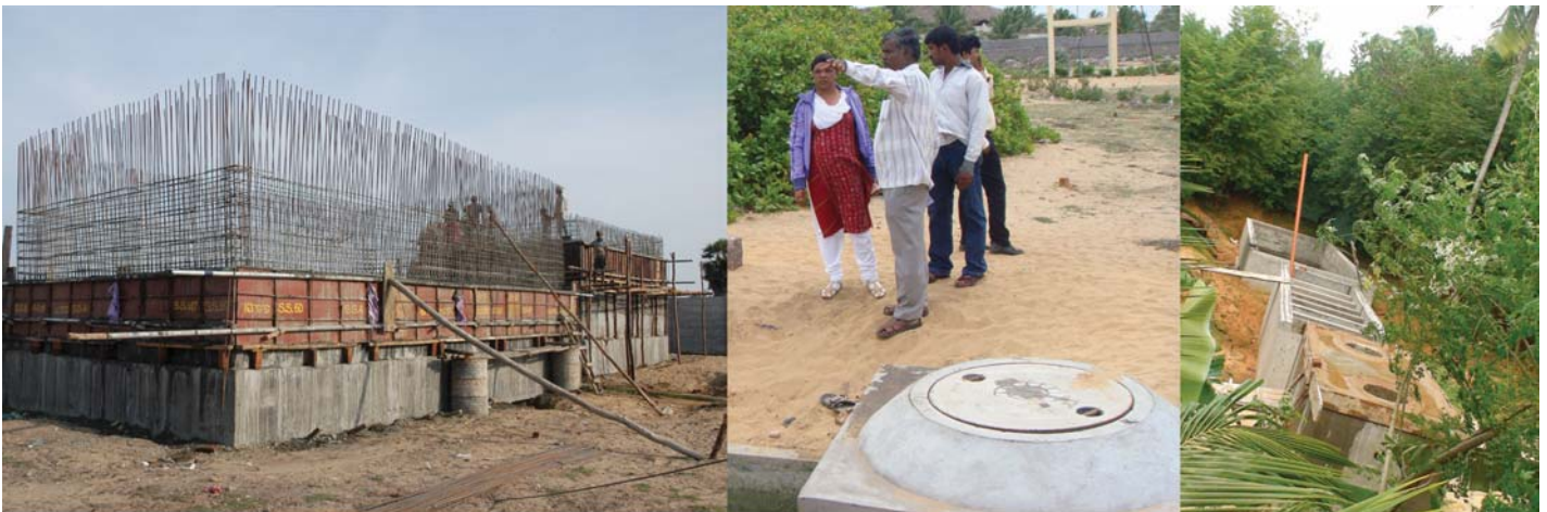
DEWATS Construction at Tsunami affected areas
