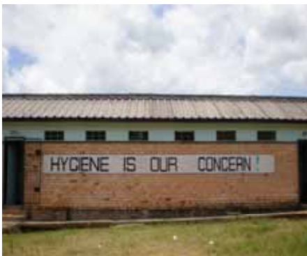
School Sanitation block in Zambia before intervention: the importance of good hygiene is already noticed.
