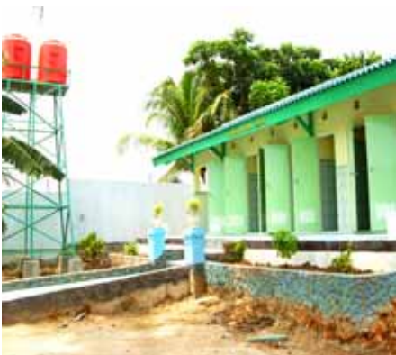
Water tanks guarantee the provision of fresh water
